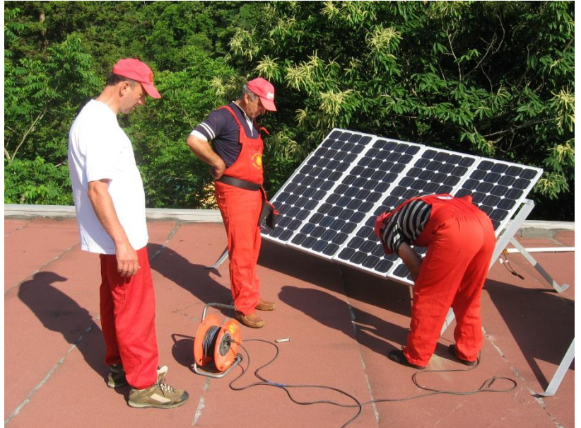
Photo by : Adjara Sustainable Association Installing Helio Systems
