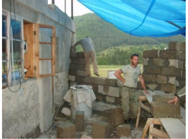
Photo by: Guram Tikanadze Svaneti Youth Center Constructing eco-guesthouse
